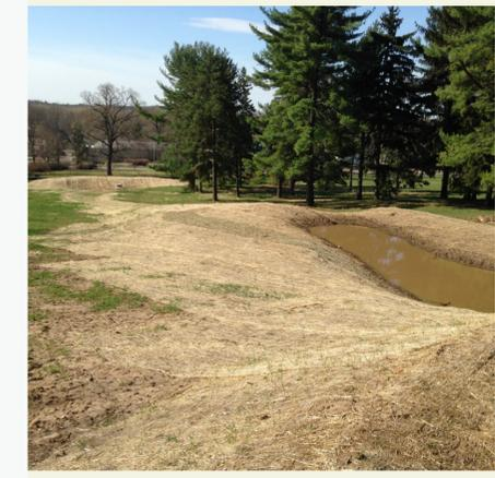
New stormwater basins hold back runoff into Warner Park and Lake Mendota. The new ponds and channel manage stormwater better than the old, while preserving historic features and views.
